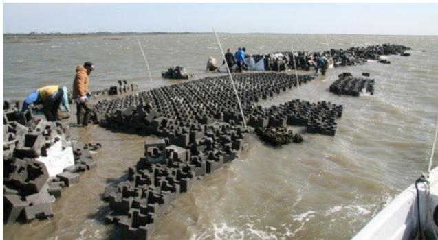
**Figure 11: Oyster Reef under Construction
