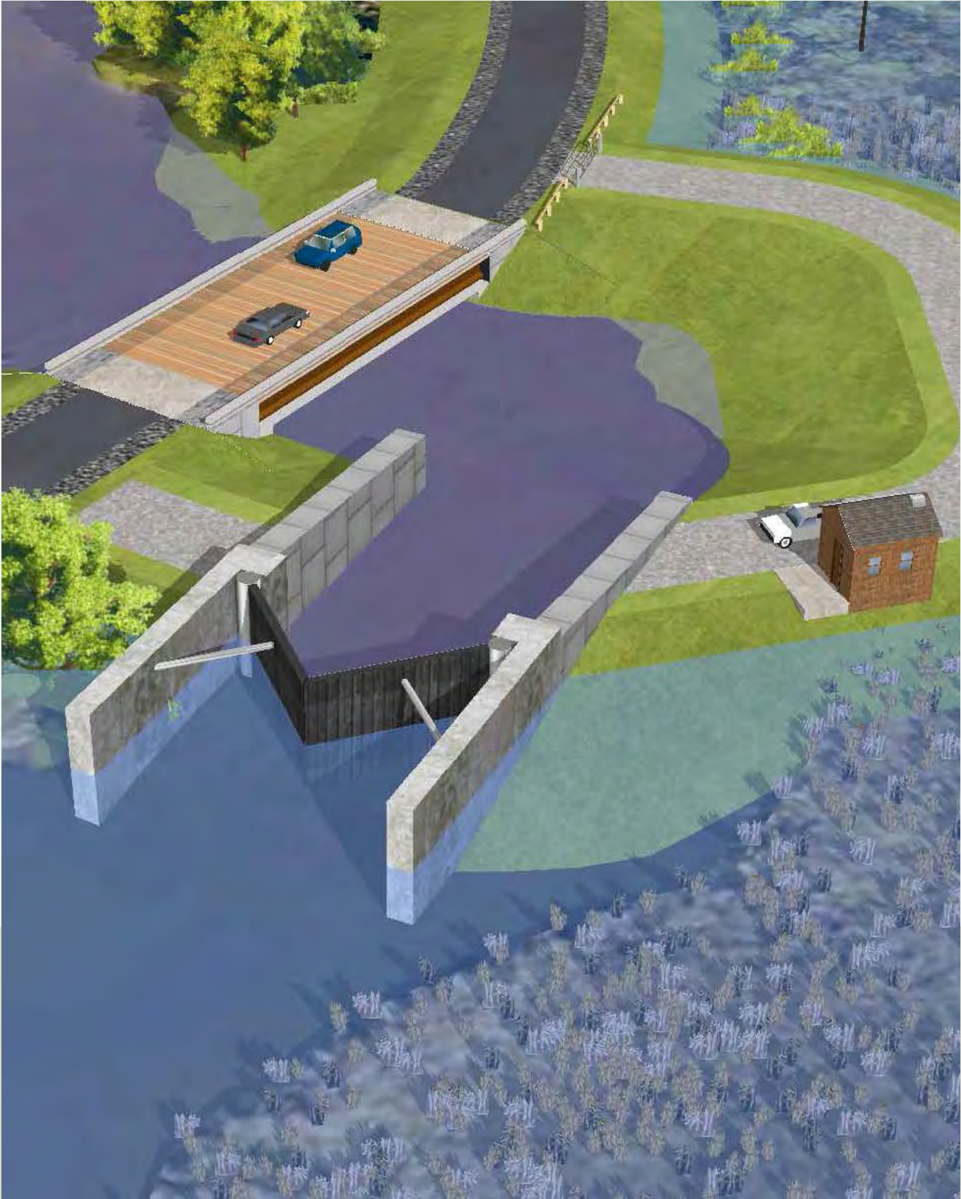
Muddy Creek Road structural protection system under flood condition (enlarged view)
